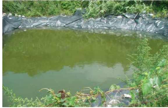
Plastic-lined retention ponds (Source: Bai, 2014)
