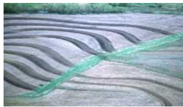
Contour terraces draining into a grassed waterway.
