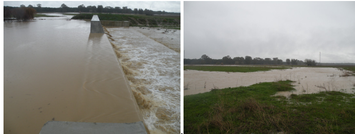
Figure 7: Flood in the Arroyo del Partido stream at 13:10 h local time on February 5 2009. Left: flow distribution at the CD1. Right: the flood flows downstream over the flood-lamination-sedimentation plain.
