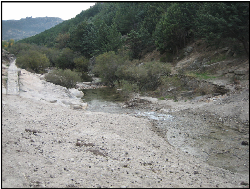
Figure 3 – Manzanares dam after the demolition
