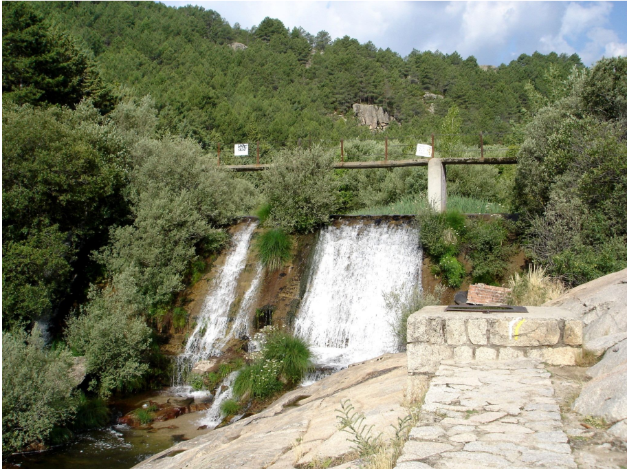
Figure 1 – Manzanares dam before the demolition
