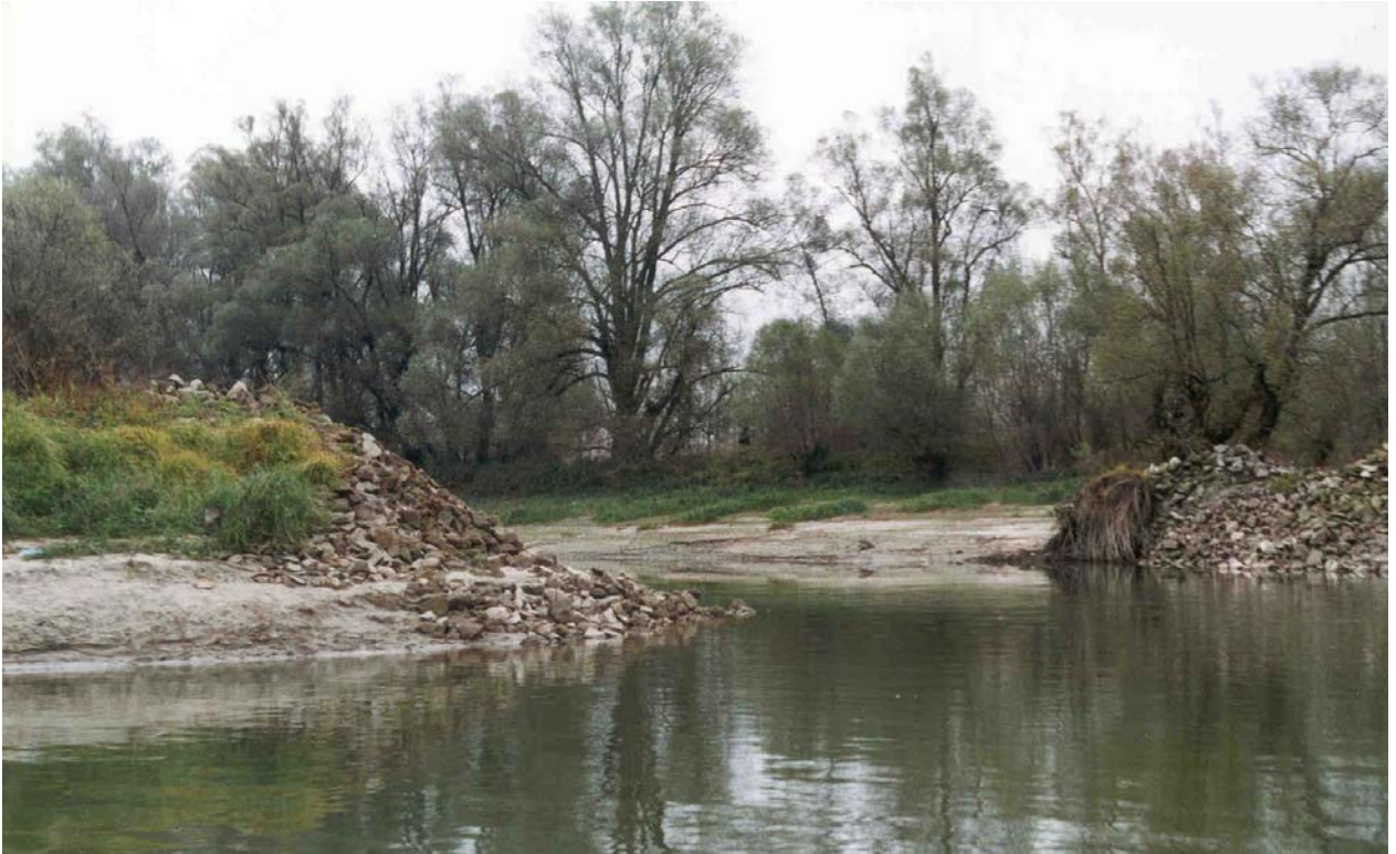
Photograph 3. The reopened rock dam
